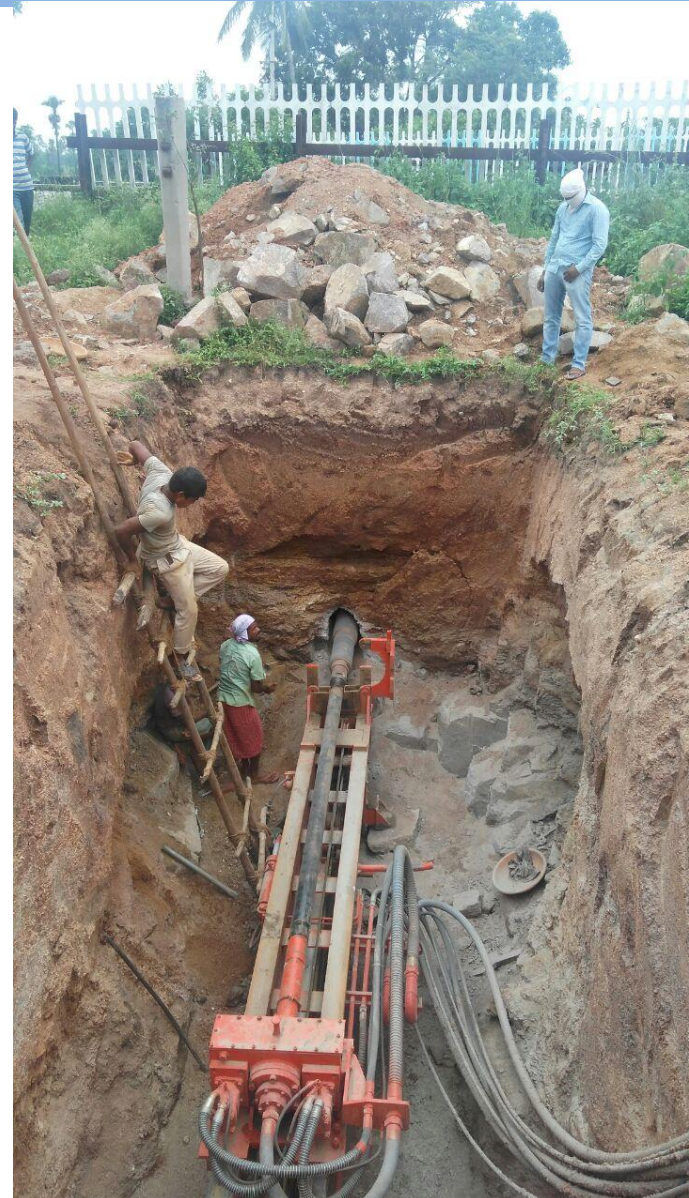
Railway crossing @ Vangapally
