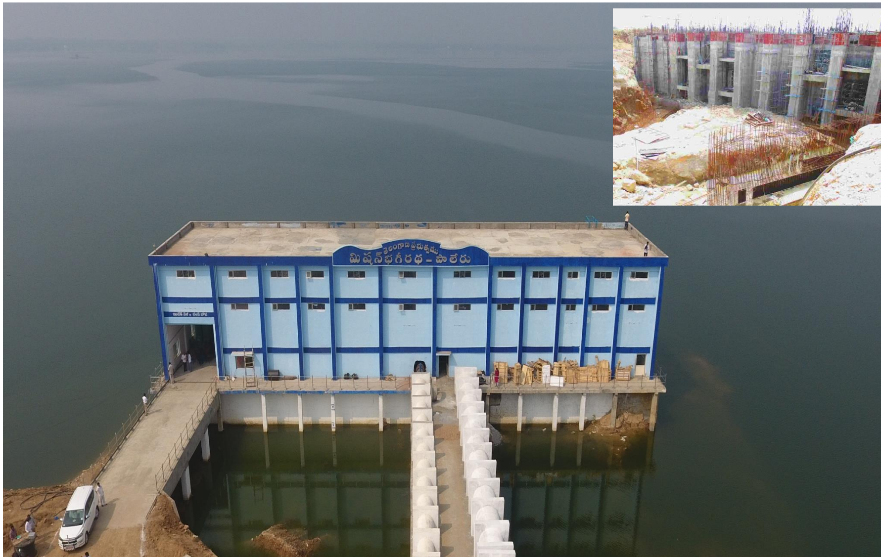
55m x 12m x 14m Intake well
